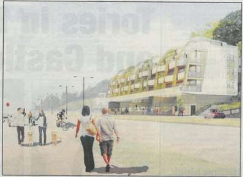
It's the new thing - how the seafront apartment block will look. Developers expect great interest
